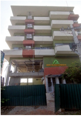
88 th Developer (Pvt) Ltd Alakeshwara Apartment (Supply & Installation of Total Fire Protection & Detection System)
