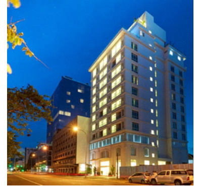
Mandaraine Hotel Colombo Annual Maintenance work - Fire Detection system
