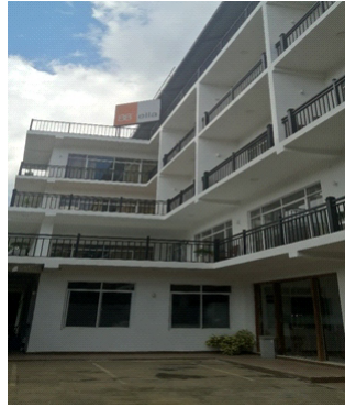
88 th Ella Project (Supply & Installation of Total Fire Protection & Detection System)
