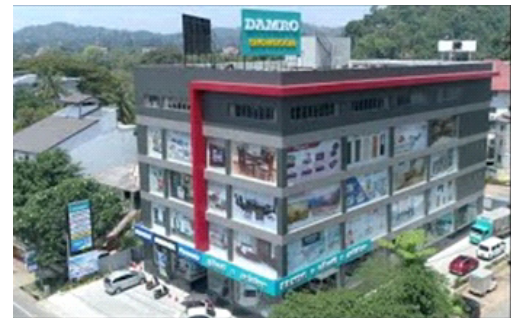
Damro Showroom Project- Ratnapura,Matara (Total Fire Protection & Detection System and Plumbing System.)
