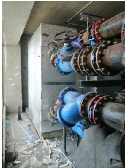
Pearl Grand Tower Hotel Project (Supply & Installation of Insulation Jacket for Heat Exchanger )
