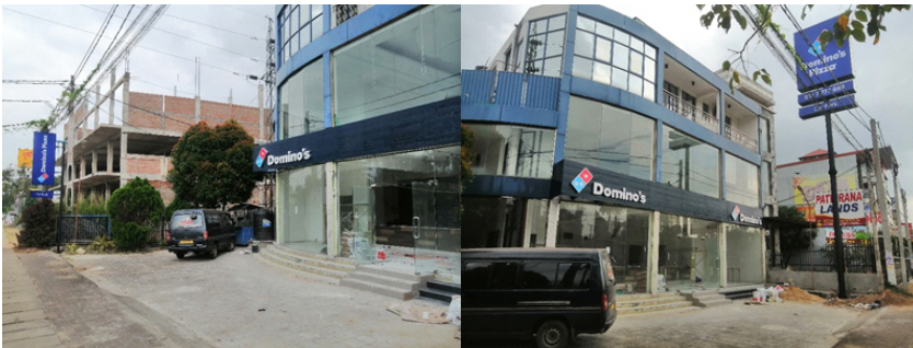
Domminos Pizza Outlets–Supply & Installation of Fire Detection & Extinguishers System & LP GAS System
