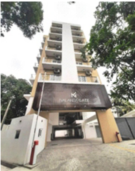
Thamaniya (Pvt) Ltd.Nalanda Gate Apartment (Annual Maintenance work of Fire & LP Gas System)
